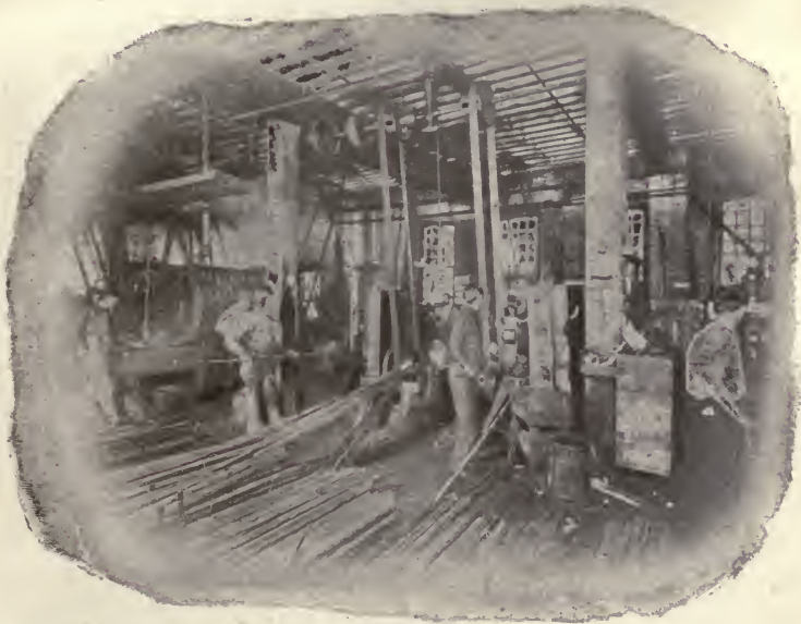
Steel Room, Cutting to Multiples.
