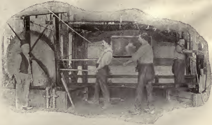
Hardening Circular Saws.
