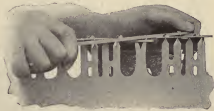
FIG. 3. FILING RAKER TOOTH
