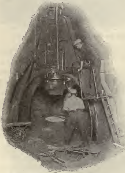
This Steam Hammer strikes a blow equal to 2½ tons.
