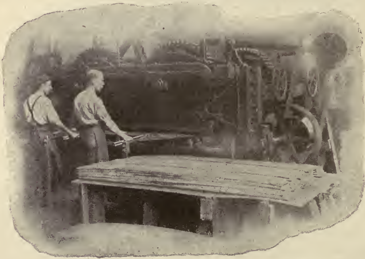
Cutting to shape.
