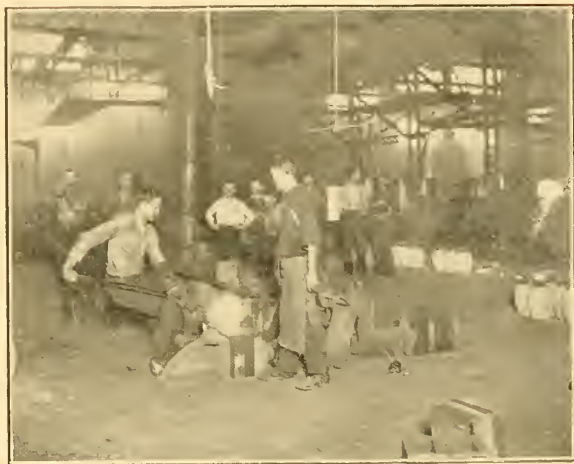
MAKING CRUCIBLE INGOTS FOR SAW STEEL
