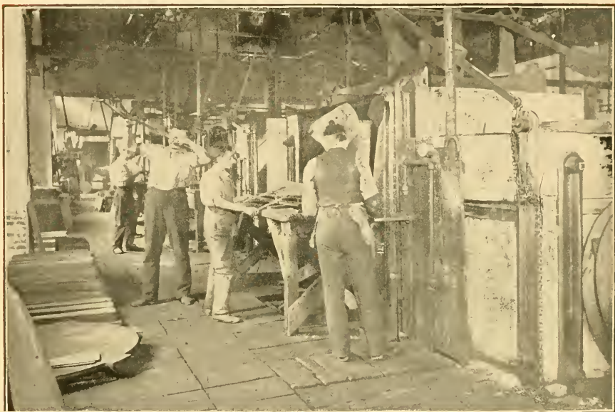
HARDENING AND TEMPERING HAND SAW BLADES
