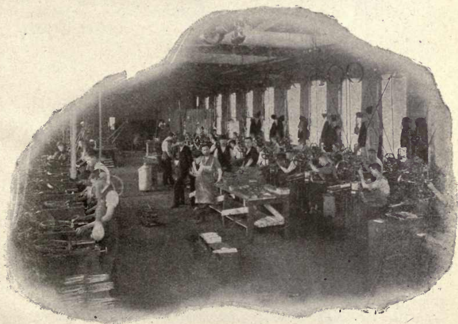
"Stripping" and "Cutting" Small Files.
