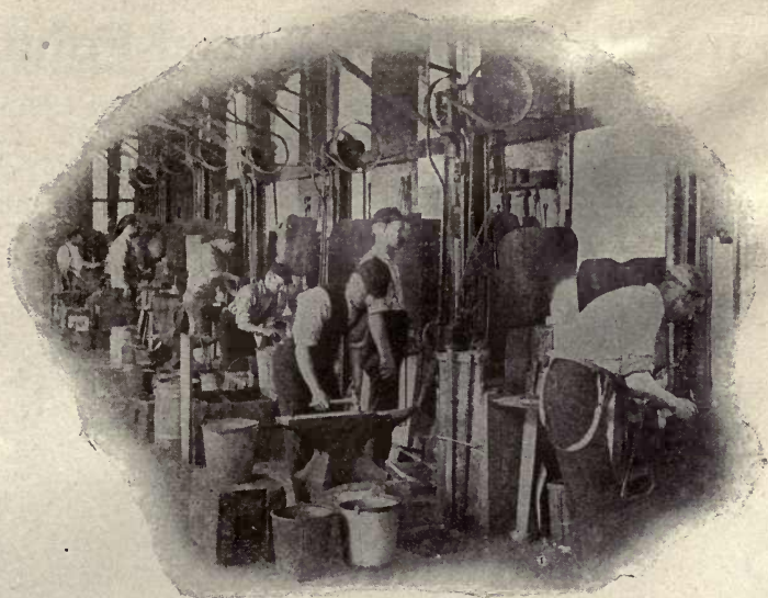
Forging Teeth for Inserted Tooth Circular Saws.
