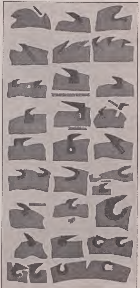
Early Types of Inserted Teeth for Circular Saws
