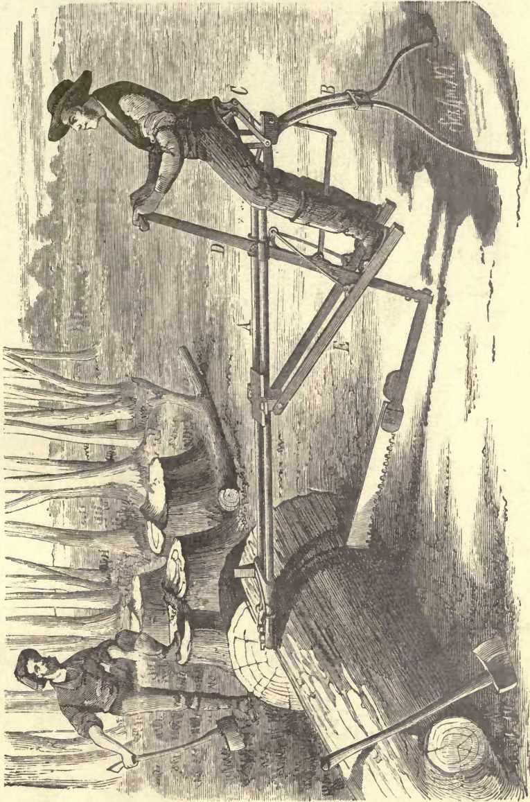
Fig. 27. Giles' Drag Sawing Machine.
