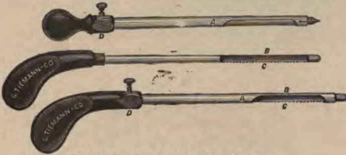
Fig. 42. Protected Rasping Saw.
