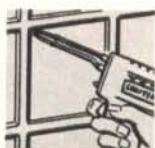
Remove old putty from window frames
