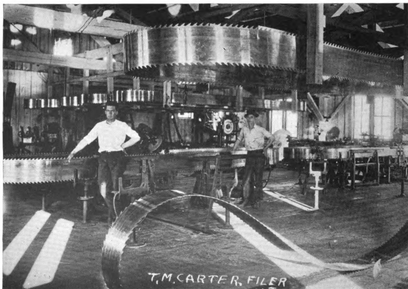
West Lumber Co.'s Filing Room, showing Disston 14-inch double-cut bands worn down to 8 inches.
