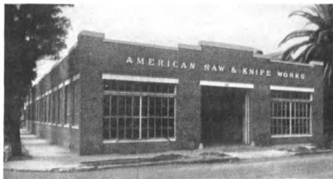
The American Saw and Knife Works. A class C building 52x140 feet, designed especially for proper light and machinery arrangement.
