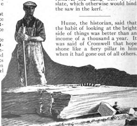
Disston Slate Saw Severing Block of Slate
