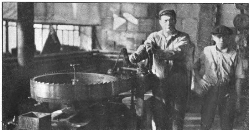
Filing room of Mengel Box Company, Jersey City, N. J. Mr. M. E. Simpson, the Co.'s filer, swaging a Disston Saw.
