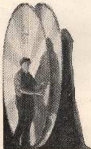
Fig. 76.—One hundred and ten inch circular saws for Western logging.
