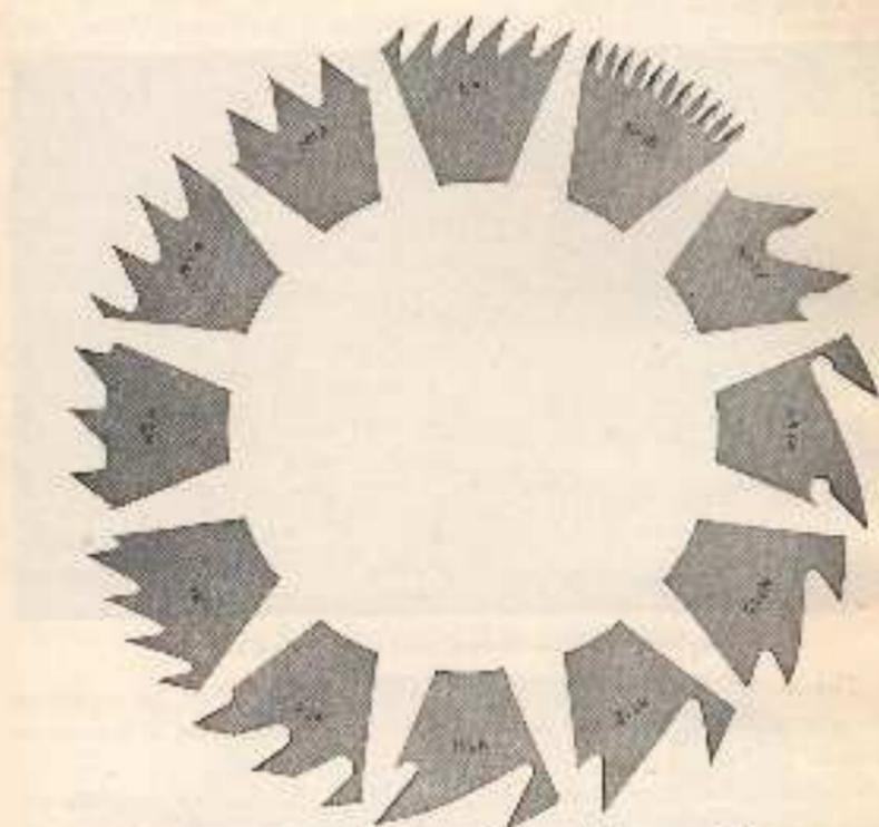
FIG. 73.—Seventeen sections of Disston circular saw teeth.
