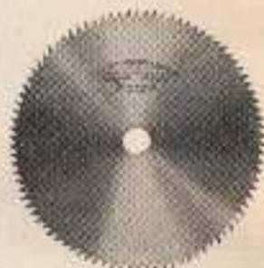
Fig. 180.—Cross-cut Circular Saw.
