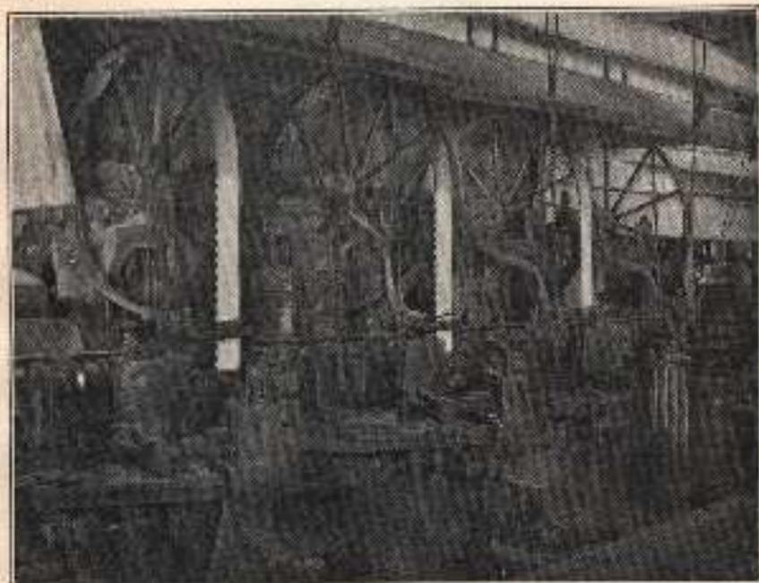
Fig. 77.—Four band gang saw in modern mill.
