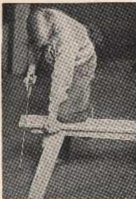
Fig. 15.—Front view of correct cross-cutting position. Note straight line of action.
