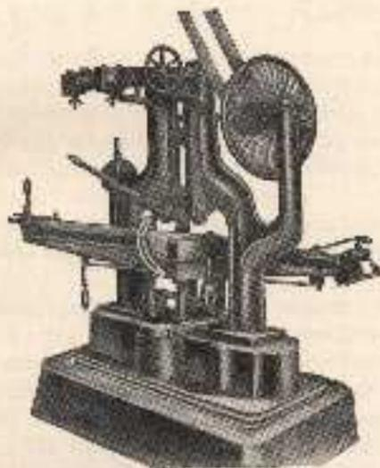
Fig. 97.—First practical file-cutting machine. Invented by E. Bernot.
