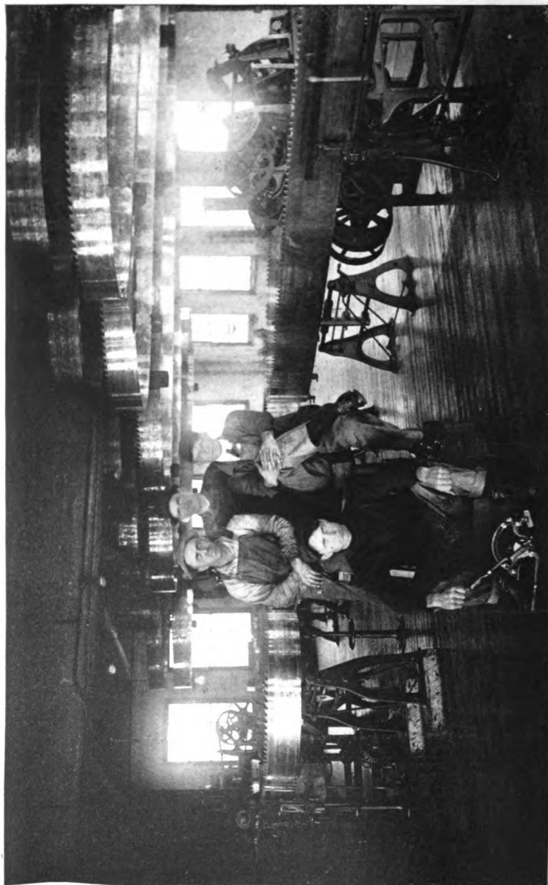
This is the Filing Room of the Dare Lumber Company, of Elizabeth City, N. C., equipped with Covell Mfg. Company's machinery, and all the band saws you see in the Filing Room are Diastons. So, except one pair, this mill has two 12-inch Band, and one 10-inch Resaw, capacity 128,000 feet, every ten hours one hundred and twenty-five thousand feet. Mr. G. Litchfield, the one in the picture who is sitting on the sawage stand with his leg crossed, is the head filer, and Mr. J. M. Barnes, who is sitting at Mr. Litchfield's feet, is the helper. The other two men in the picture are the superintendent and millwright. Mr.
