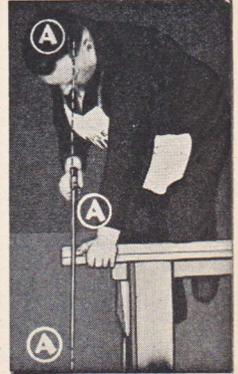
Fig. 10—Correct position for straight sawing.
