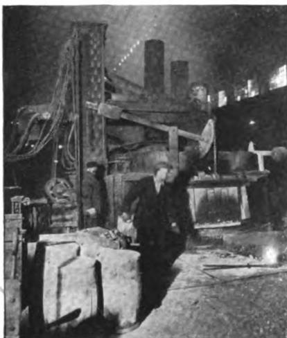
Taking Laboratory test sample from electric furnace
