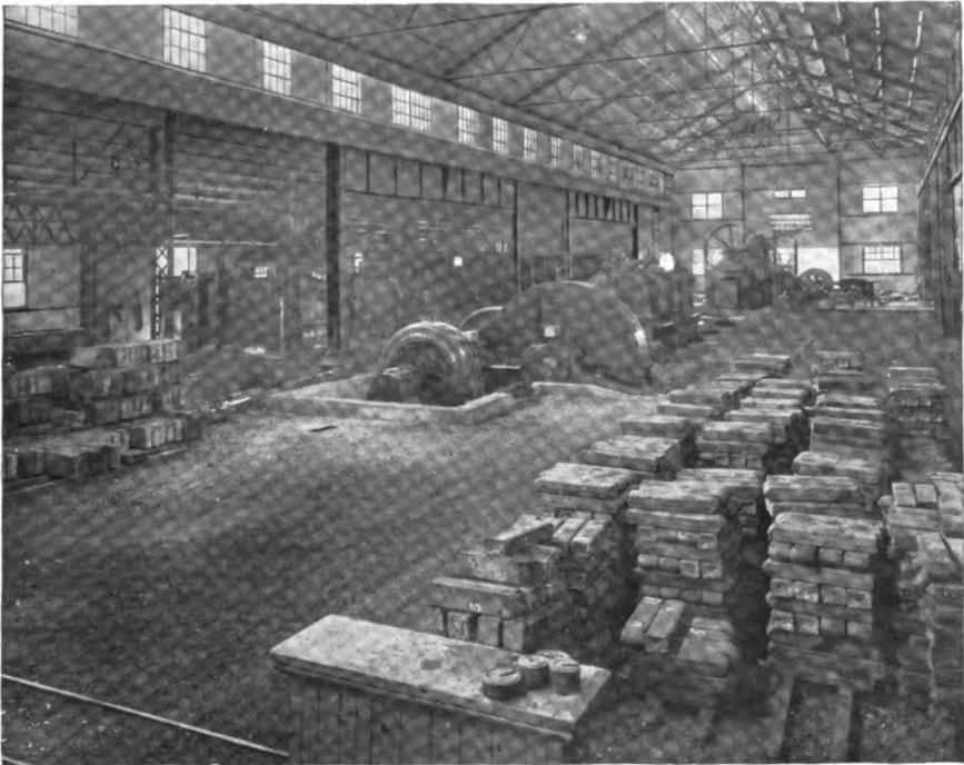
Cogging Mill with ingots ready to reheat
