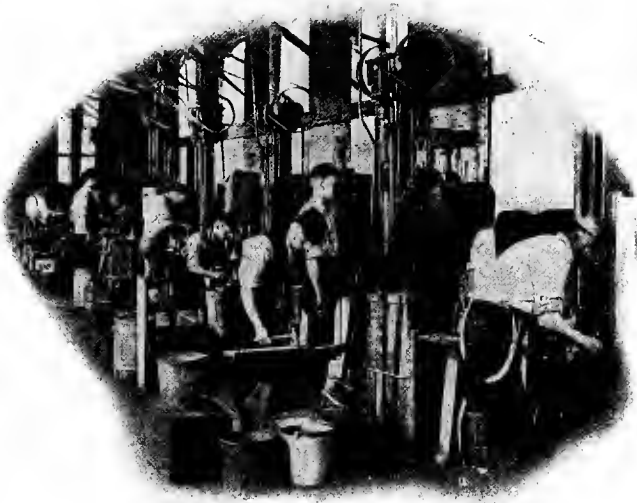
Forging Teeth for Inserted Tooth Circular Saws.
