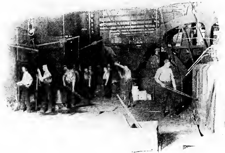
Rolling Hand Saw Plates.
